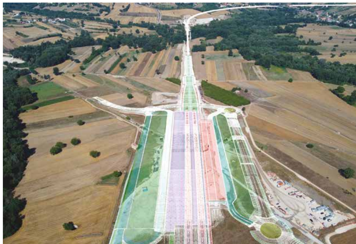
A fianco / Next to Progettazione in BIM della linea AV/AC Napoli-Bari. BIM design of the Naples-Bari high-speed/high- capacity line.
